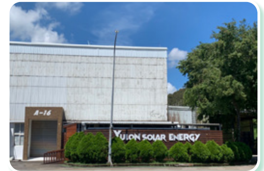
Solar Power and Energy Storage Demonstration Site
