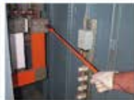
▲ Training on the safety of high voltage power line maintenance & inspection
